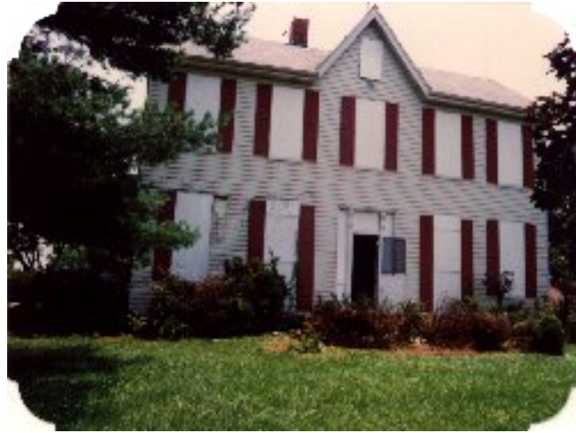
Draper Property in 1996 before repairs
